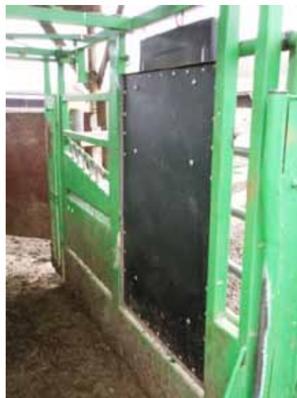
Insertion of a composite panel (Jalogny)
