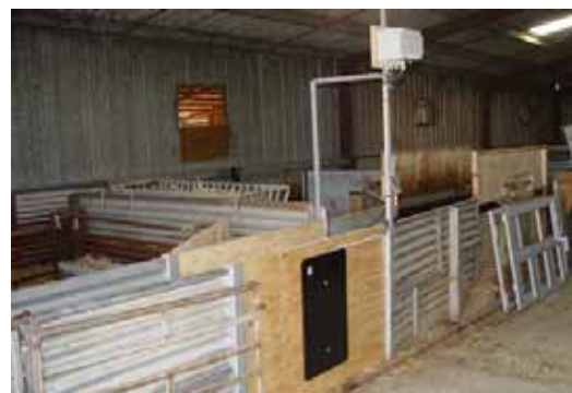
Integration of a wooden panel containing a Réseumatique antenna into a working chute (CAVEB, Deux-Sevres).
