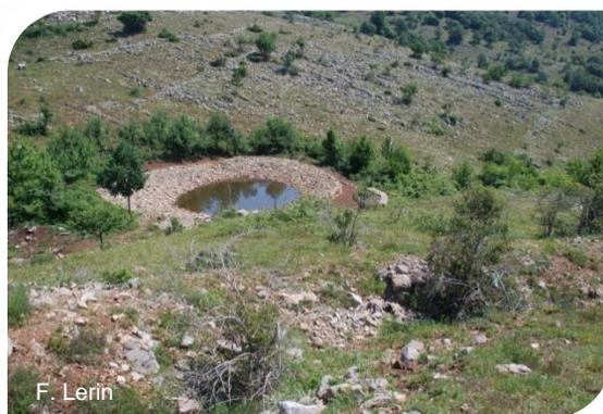
A lavogne was recently built in Cahan. The stock farmers do not use it because it was badly designed and badly built (the plastic waterproofing was made from an unsuitable, fragile material which was quickly torn. A stock farmer explains: *“They issued a call for tender but no one consulted us... they would have been better advised to give us the money and we would have done something useful for our farms.”*
